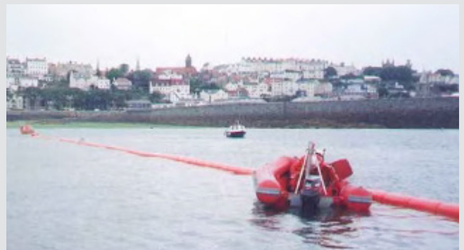
4. Small work boats are used to tow and position the cable.
