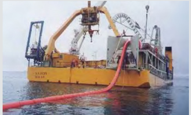
3. The HVAC cable and SeaSerpent being deployed at Havelet Bay.
