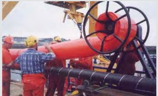
2. SeaSerpent being attached to the HVAC cable showing Seaflex manual brake RDS.
