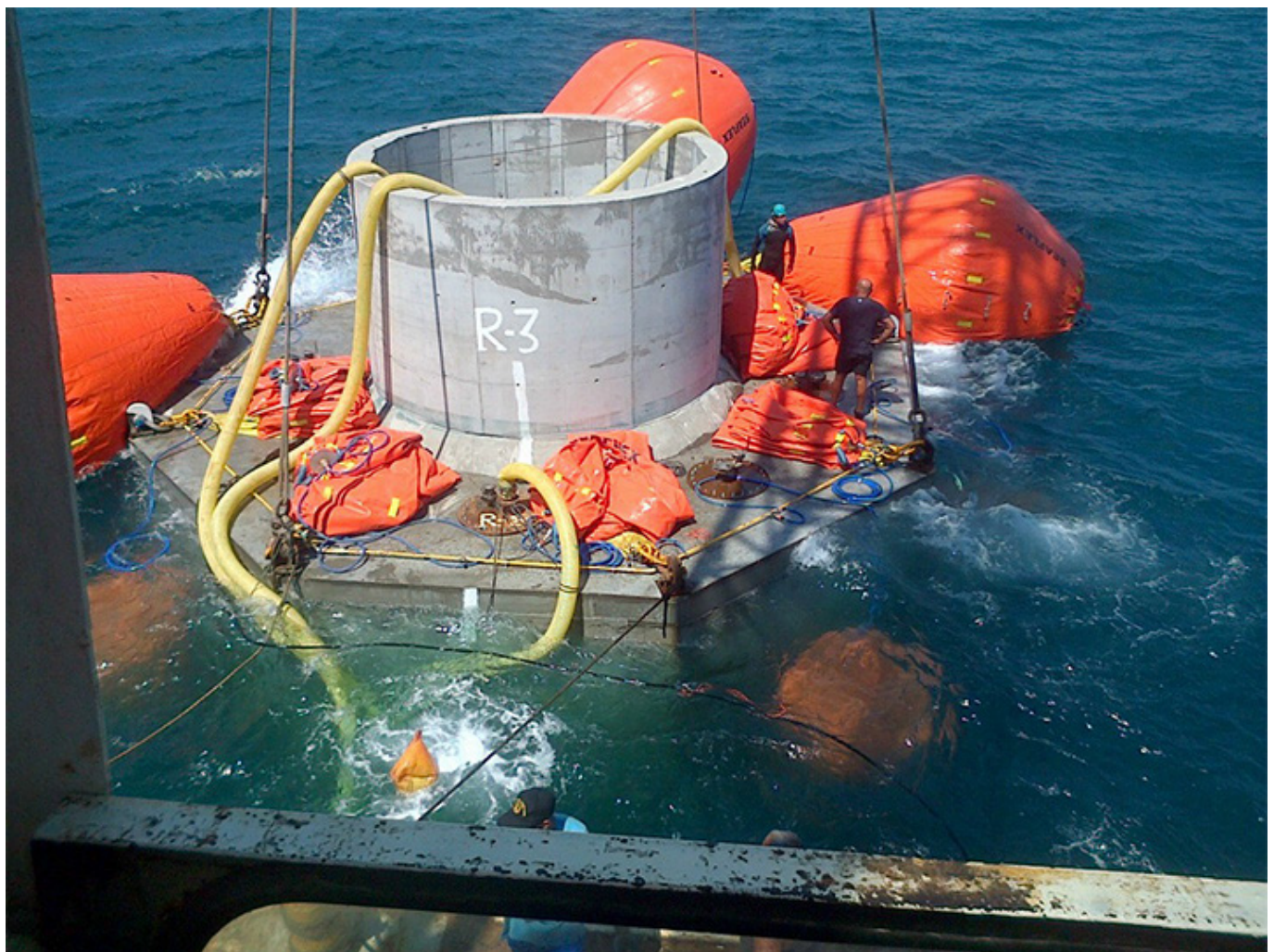
Sinking of Intake Tower (note submerged lower tier of buoys as upper tier is inflated).
